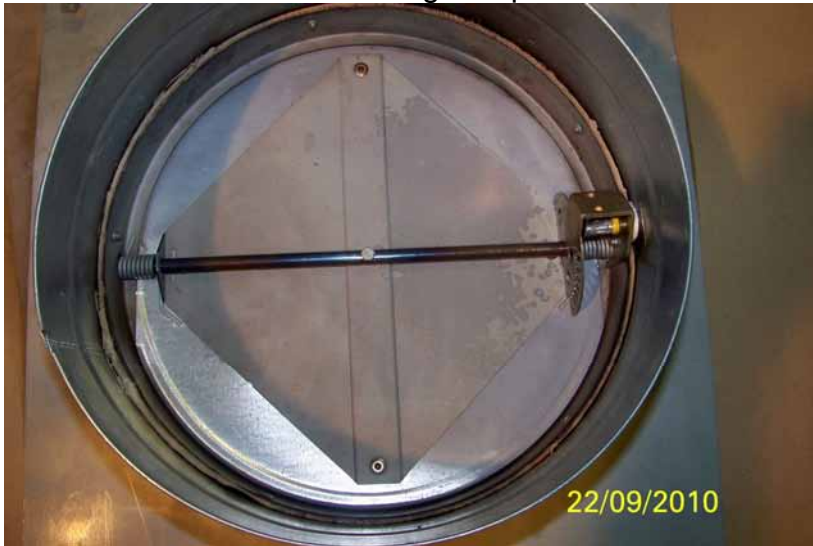
FTP 11 After 25 min's showing damper blade condition with furnace at 812°C
