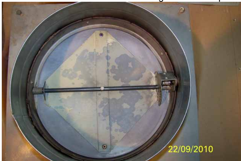
FTP16 Fire test after 50 min's showing 315 dia damper at 883°C
