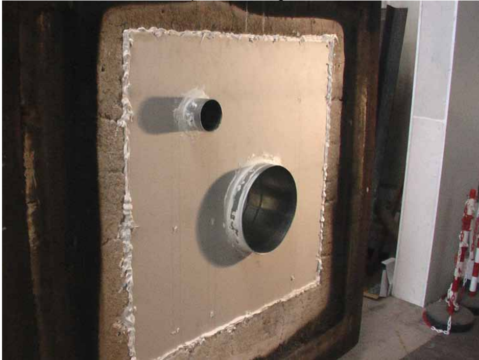
FTP 5 Inside Face of wall prior to fitting to furnace.
