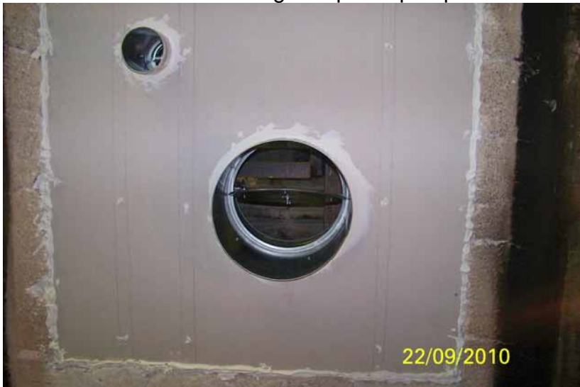
FTP 6 Internal face showing dampers open prior to starting the test.
