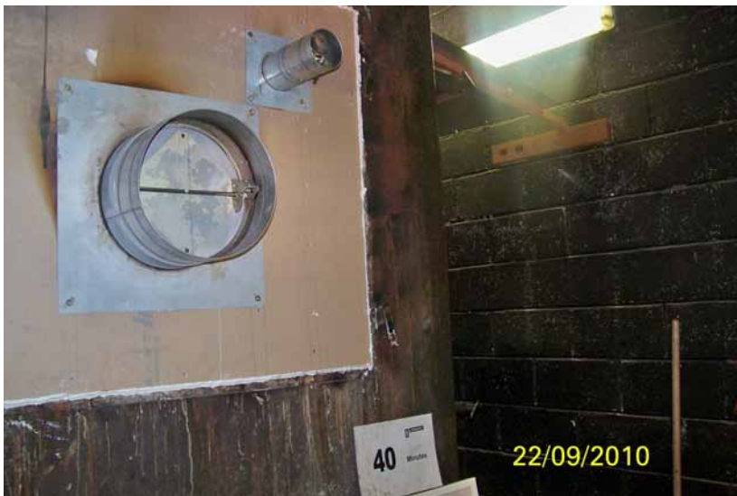
FTP 14 Fire test after 40 min's
